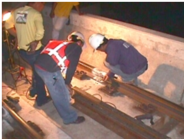
MAGNETIC PARTICLE TESTING AND ULTRASONIC TESTING OF RAIL THERMIT WELDS
